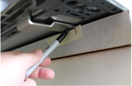
4. Remove oven and place brackets at the desired location.
